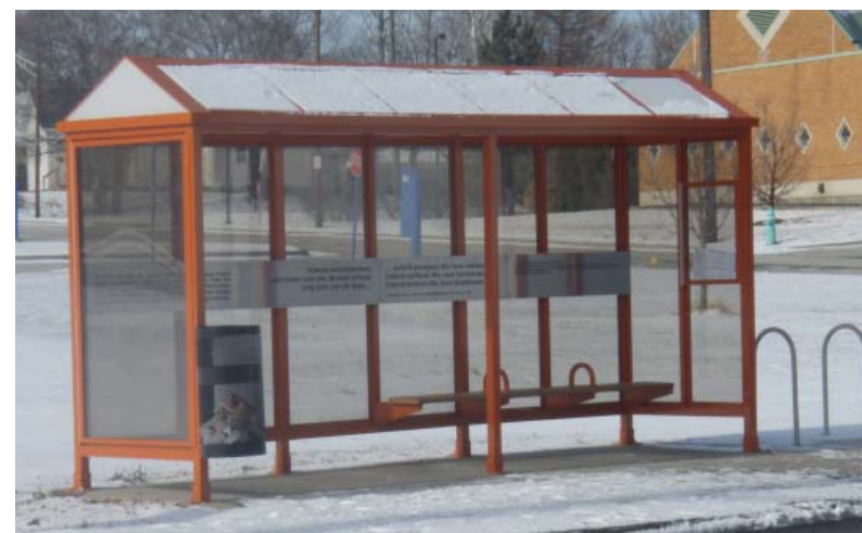
Example of enhanced bus shelter with bike racks Martin Luther King Blvd. Streetscape (designed by SKA)
